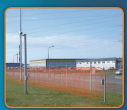
Microwave barrier with narrow detection zone can be used when customer want to have as much utilizable space as possible.
